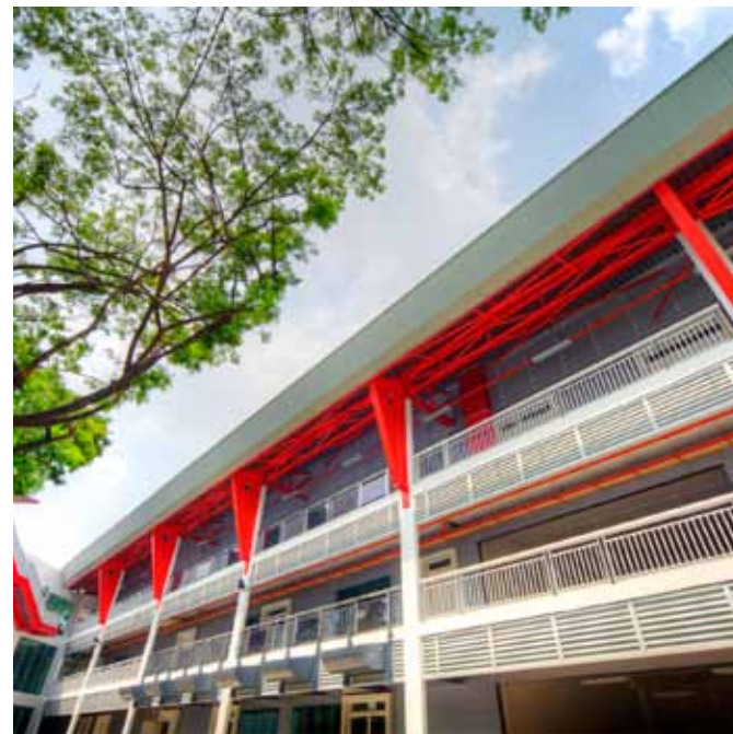
Zero Energy Building @ BCA Academy - the first existing building in Southeast Asia to be fully retrofitted with green building design features and technologies. It is a testbed for innovative building solutions applied at the systems level to achieve net zero energy consumption, e.g. built-in photovoltaic panels, low-emissivity glass and solar chimneys.
